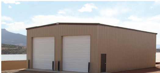
U.S. Corp of Engineers Abiquiu, NM
